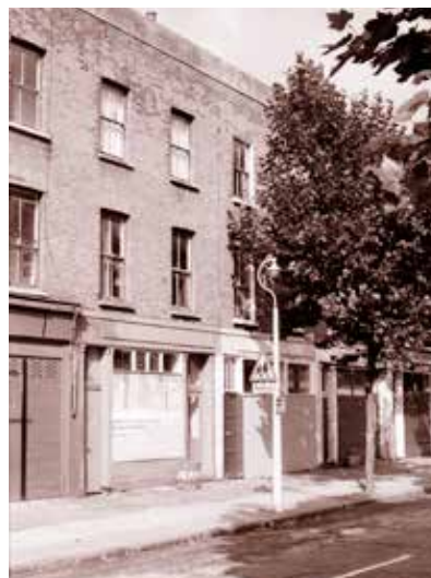
Far left Boarded-up houses on Campbell Road, E3, awaiting repairs. Acme Studios (1974)
