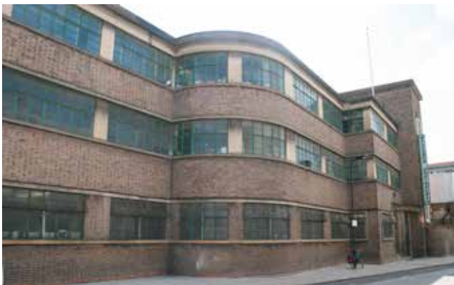
Orsman Road, N1 – purchased 2000. Acme Studios (2010)
