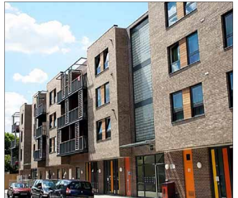
Atelier Court in E14 offers 21 Acme studios, called Leven Road, which are built into the development's ground floor. For more details, call Acme on 020 8981 6811
