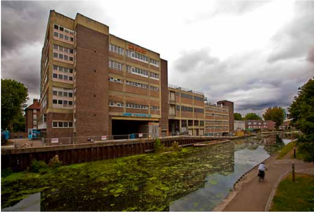
The Lesney Matchbox Toys Factory before demolition work began. Photo: Greg Goodale (2009)
