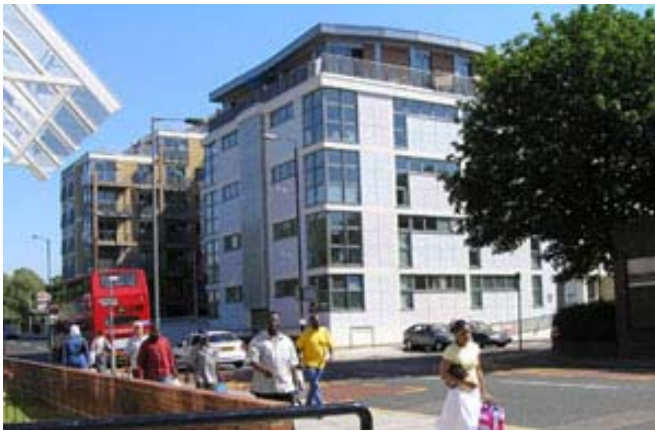
The Galleria Studios, Peckham, London, SE15
