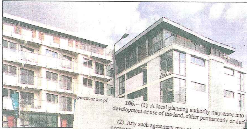
Barratt had to build 47 artists' studios as part of the Galleria, above - thanks to section 106, right.
